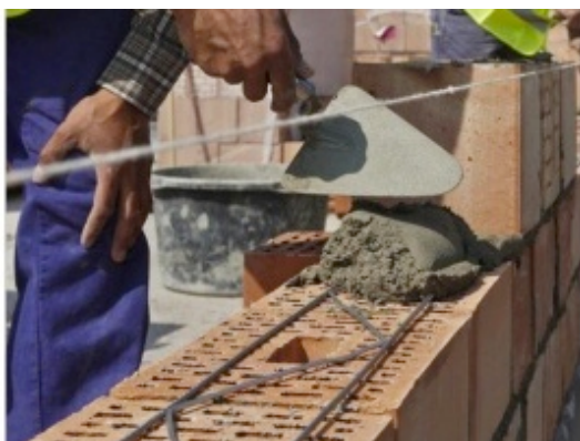
Figure 2-17. Armatures horizontales 15
