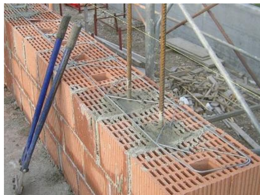
Figure 2-18. Armatures verticales 16
