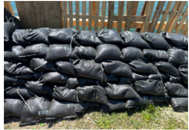
Abb. 22: Sandsacksystem (BABS)
