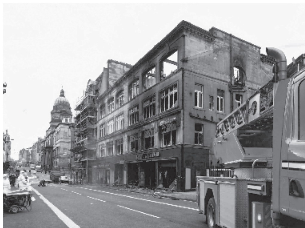
Fig. 3: Fire at South Bridge in Edinburgh
